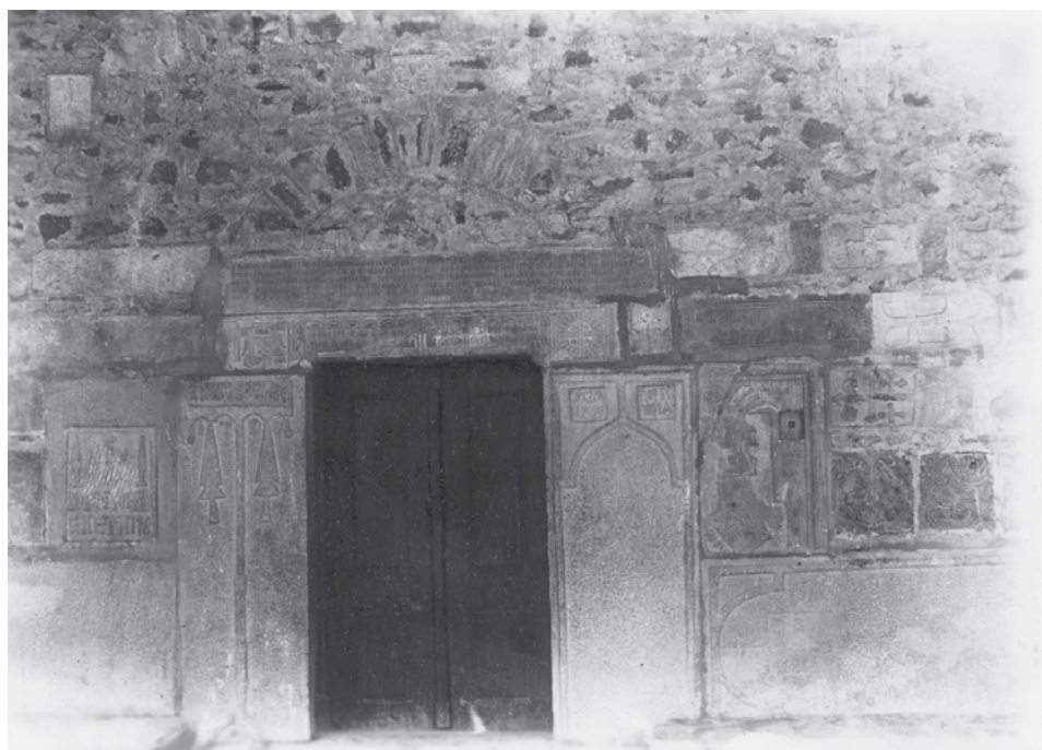
Fig. 2. Detail of the southern wall of the church prior to the removal of the carved elements. Archive of the Institute of Archaeology
