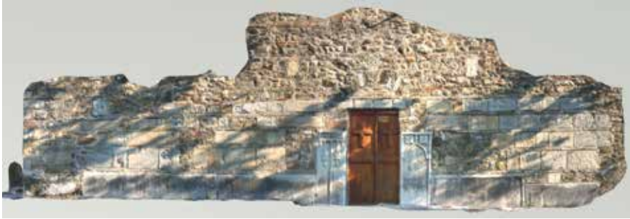
Fig. 3. Actual view of the southern wall of the church with the mayor concentration of the sculptural elements
