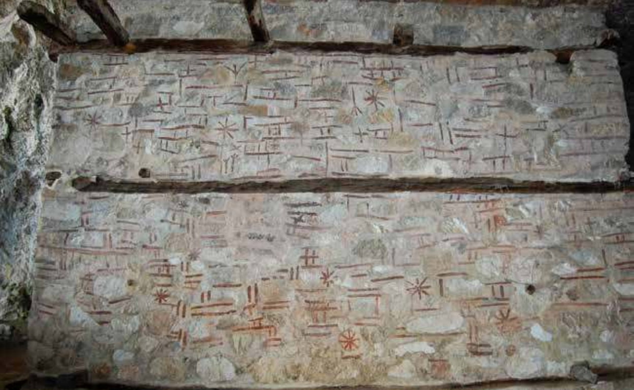
Fig. 5. The southern façade with painted motives
